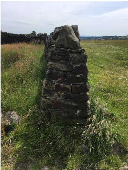
A dry stone wall in section, showing the way it was constructed
